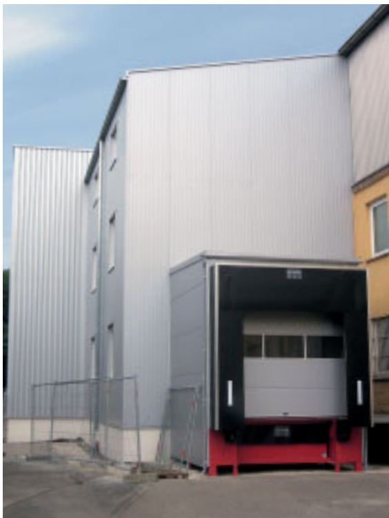
Hallenbau in Günzburg
